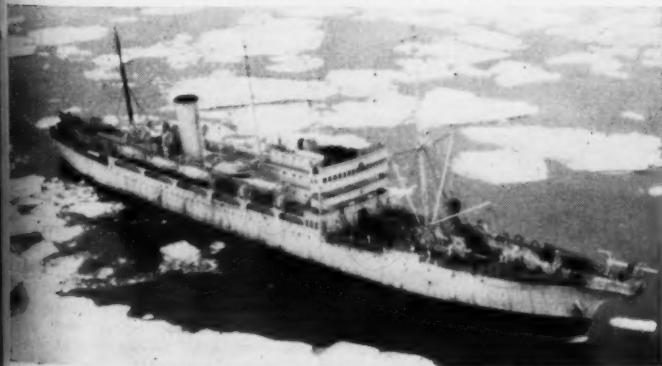
BMEWS SUBMARINE CABLE is laid by HMS Monarch in the remote, ice-choked ocean north of the Arctic Circle. Western Electric was assigned the responsibility for development and construction of the rearward communications for the Ballistic Missile Early Warning System.
